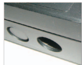
Simple electrical entries
